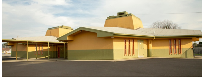
Typical classroom building at Lake Elementary School
