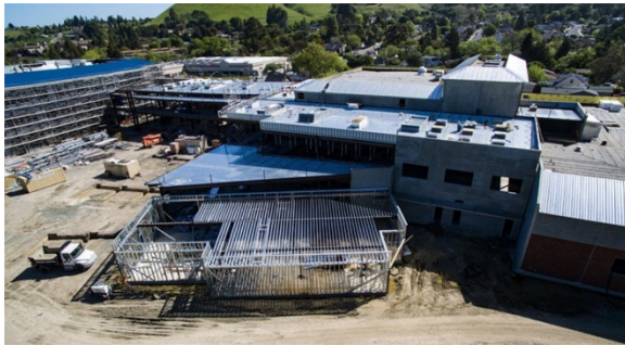
Pinole Valley High School Building A
