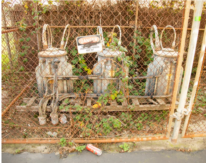
Electrical Transformers at Lake Elementary School
