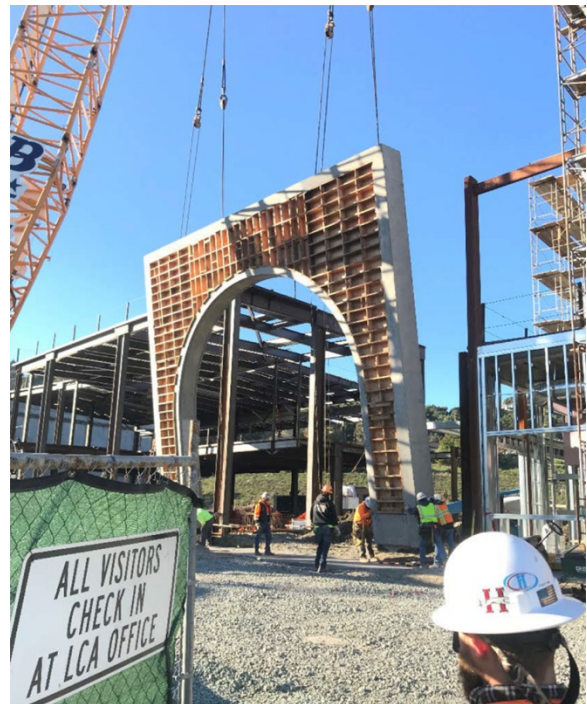
The 'face' of Pinole Valley High School--the arch--being erected
