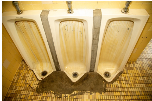
Lake Elementary School urinals in need of an upgrade
