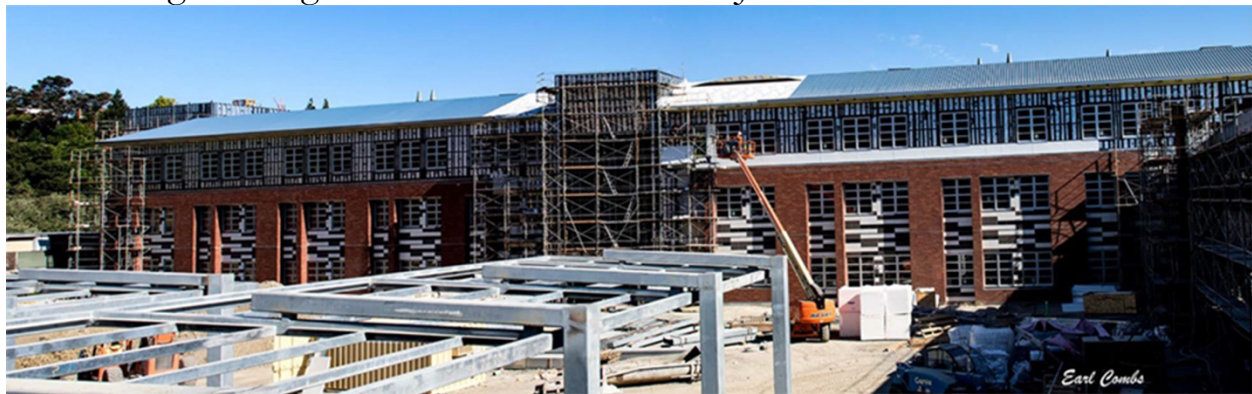
Pinole Valley High school Building D
