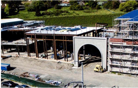
Pinole Valley High School along Pinole Valley Road
